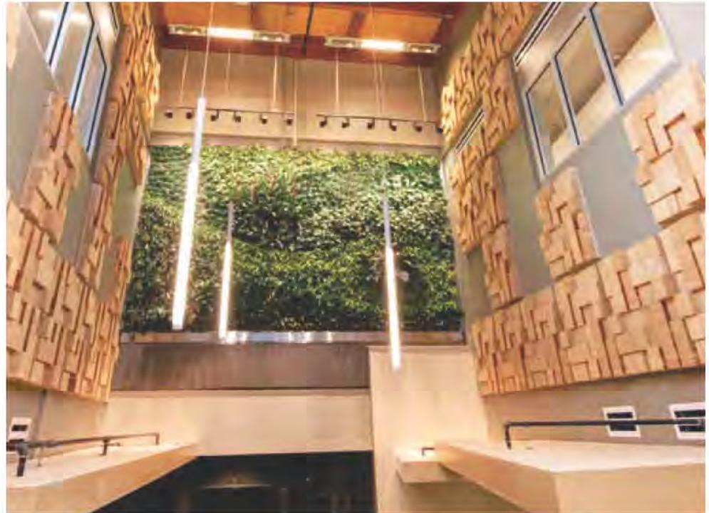
Safeway store on the site), increased insulation, high albedo white roof, exterior living wall for reduction of solar gain and an interior living wall for air purification.
